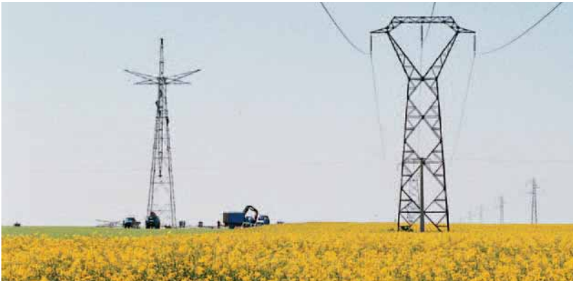
Opposite, Raising a pylon without a crane in a rapeseed field.
